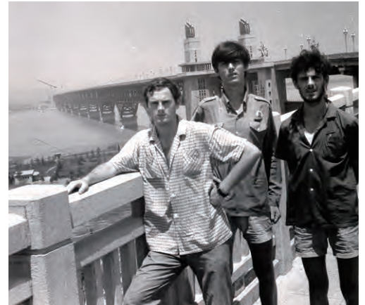
From left: Paul, Michael and Carl on the Nanjing Yangtze River Bridge in 1971
